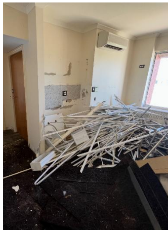
Demolition of old cabinetry
