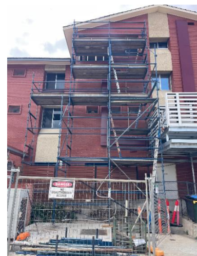
Preparations to repair the wall after the removal of the external lift.
