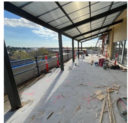
Balcony works underway
