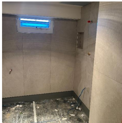
Completed tiling in ensuites
