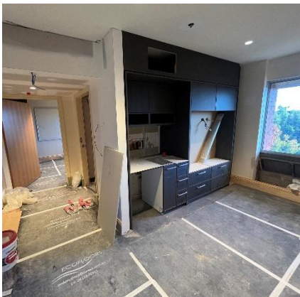
Cabinetry installed in resident suites
