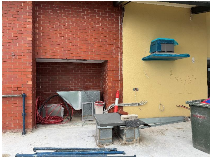
Alfresco BBQ area under construction
