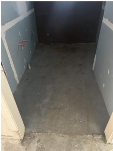
Floor screed in ensuites
