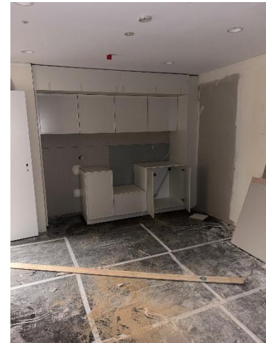
New family room cabinetry installation
