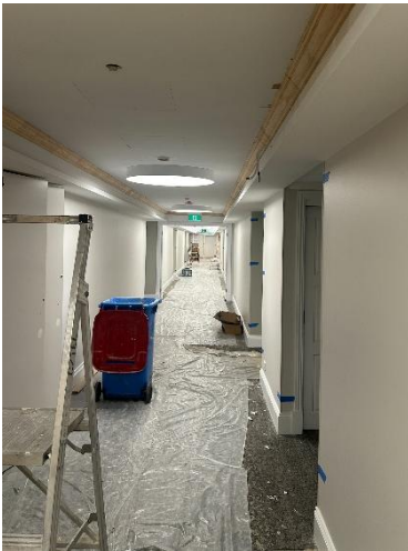
Corridors under construction
