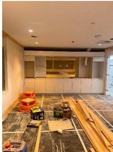
Servery for the new dining room
